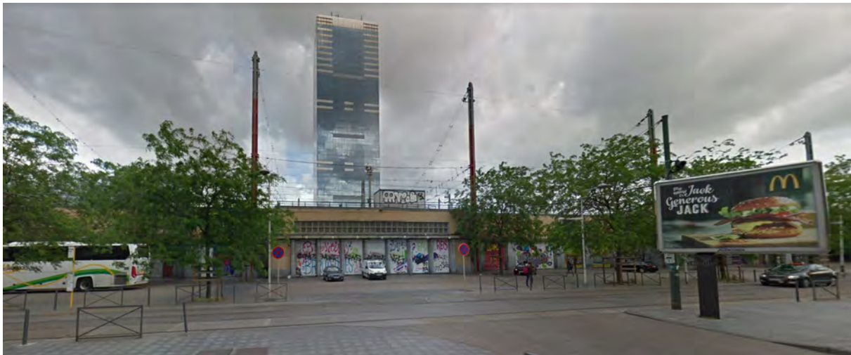
Figure 33 : Vue de la place Constitution (Google Street View, 2017)
