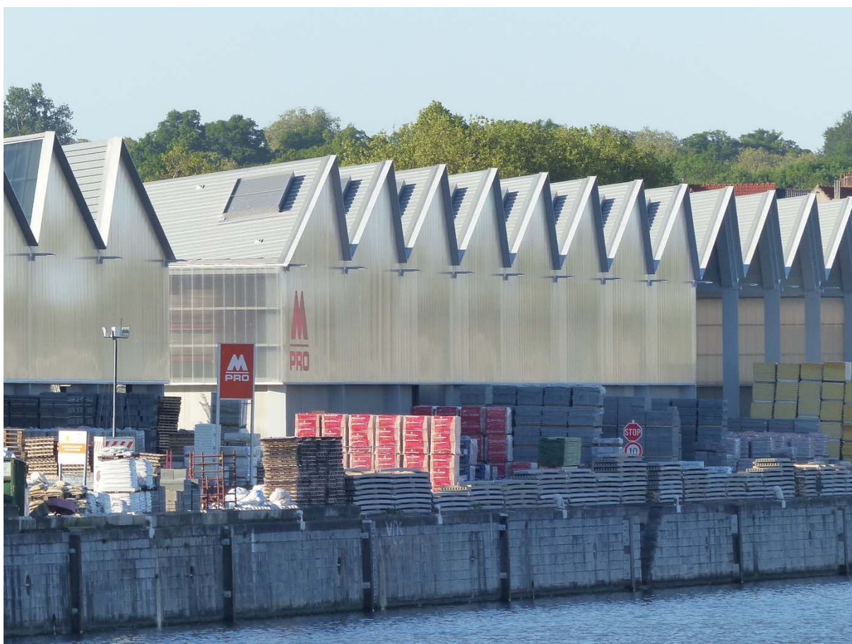
Bouwmaterialendorp, Vergotedok, Tetra architects
