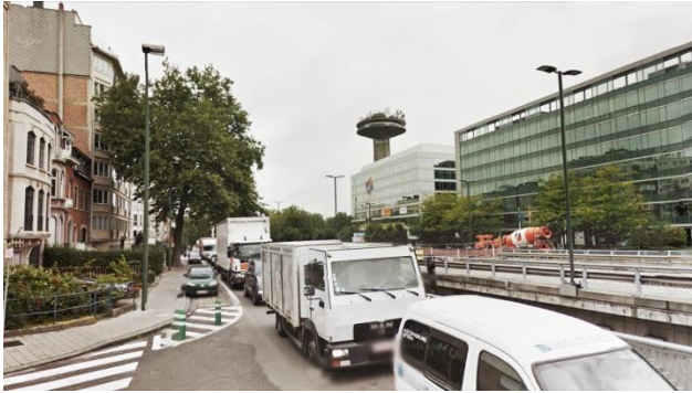
Situation existante - Boulevard Reyers
