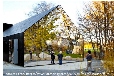
↑ MLRP architects, Mirror house, Copenhagen I Kopenhagen
