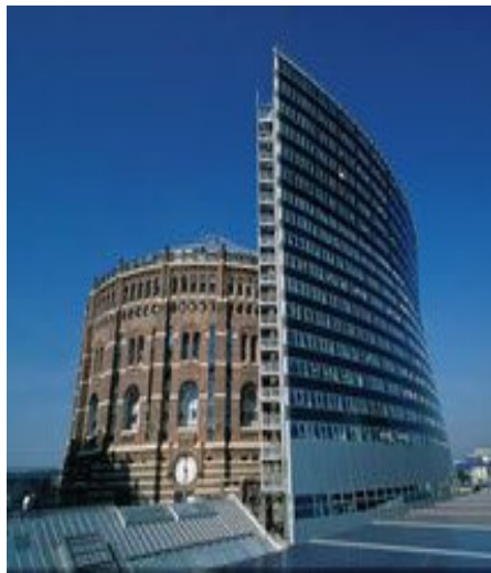
Zubau Studentenheim Gasometer
